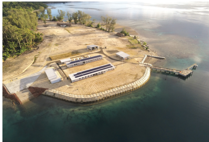
The completed Western Border Outpost at Lofung South in Shortland Islands, Western Province
