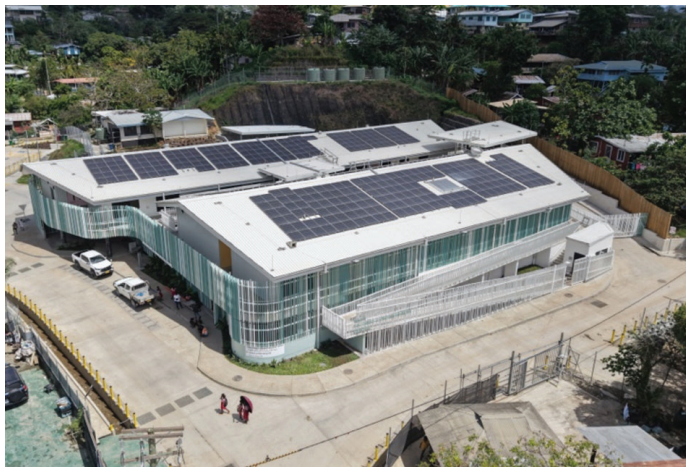
The completed Naha Birthing and Urban Health Centre
